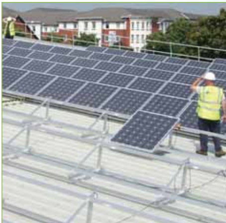
Installing the solar photovoltaic panels on 53 Degrees
